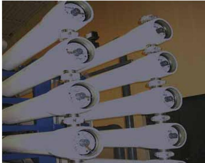
FIG. 13.5 Picture of connected multiport pressure vessels (courtesy Protec Pressure Vessels).
