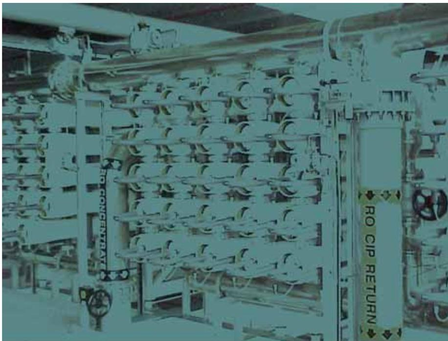
FIG. 13.6 Picture of a membrane unit with multiport pressure vessels.
